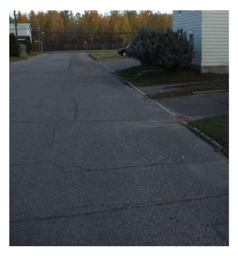
PQI=0 - 40 (POOR) Extensive moderate to severe cracking Extensive Alligator or Edge Cracking Potholes or poor patches Poor ride quality
