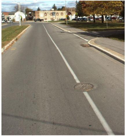
PQI = 60-80 (GOOD) Localized slight/moderate linear cracks Little to no alligator cracking present No rutting or distortions Fair to good ride quality
