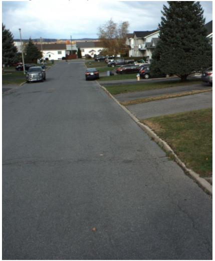
PQI=40-60 (FAIR) Extensive slight/moderate linear cracks Localized alligator/edge cracking Fair ride quality
